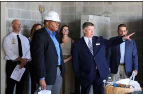
Dr. Jeremy Johnson points out some key features of the new 6-12 school currently under construction to Superintendent Green.
