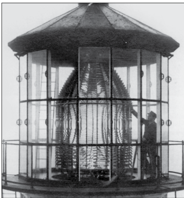
A first-order Fresnel lens similar to the Cape Hatteras Lighthouse lens, Point Reyes Lighthouse, California. Photo: U.S. Lighthouse Society
