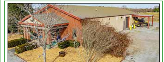
ORIENTAL – 4,000 hsf commercial, fully-insulated. Reception, conference room, 2 offices. Carrier 2.5 ton heat pump for office area, 2 5-ton HVAC systems for warehouse. Attic, 208 3-Phase 200 amp elec system. Ingersoll Rand 200 PSI air compressor. Fabrication equipment does not convey. OFFERED AT $ 575,000
