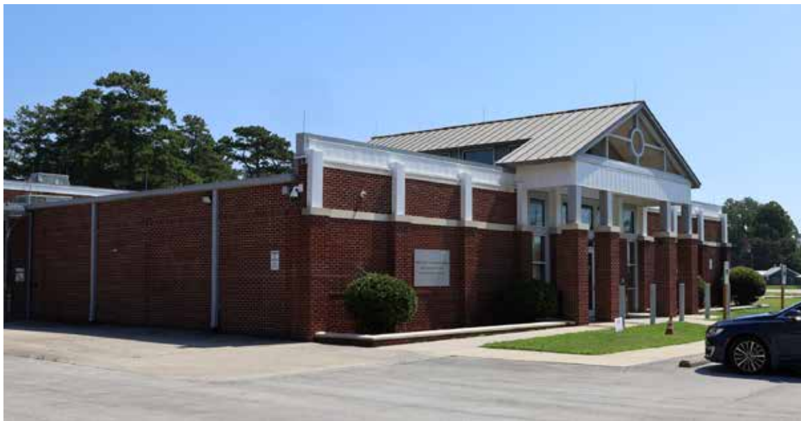
The Pamlico County Sheriff's Office and Detention Center.
