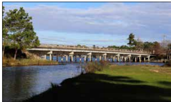
Dawson Creek Bridge
