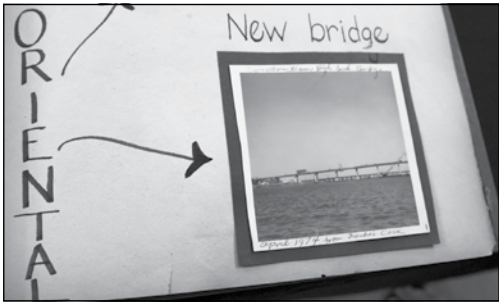
Photograph of the Bob Scott Bridge under construction from April of 1974.
