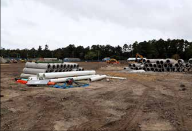
Outside, work continues prepping the area in front of the new school for installation of the drainage system and paving.
